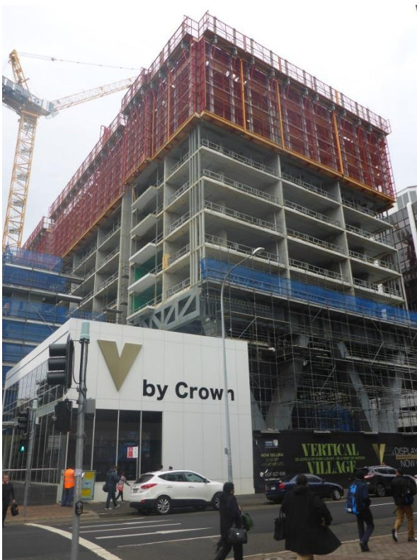
PICTURE 15 – V BY CROWN SITE AT THE SOUTHWEST CORNER OF MACQUARIE AND MARSDEN STREETS, AT 134–140 MARSDEN STREET ARCHAEOLOGICAL SITE
