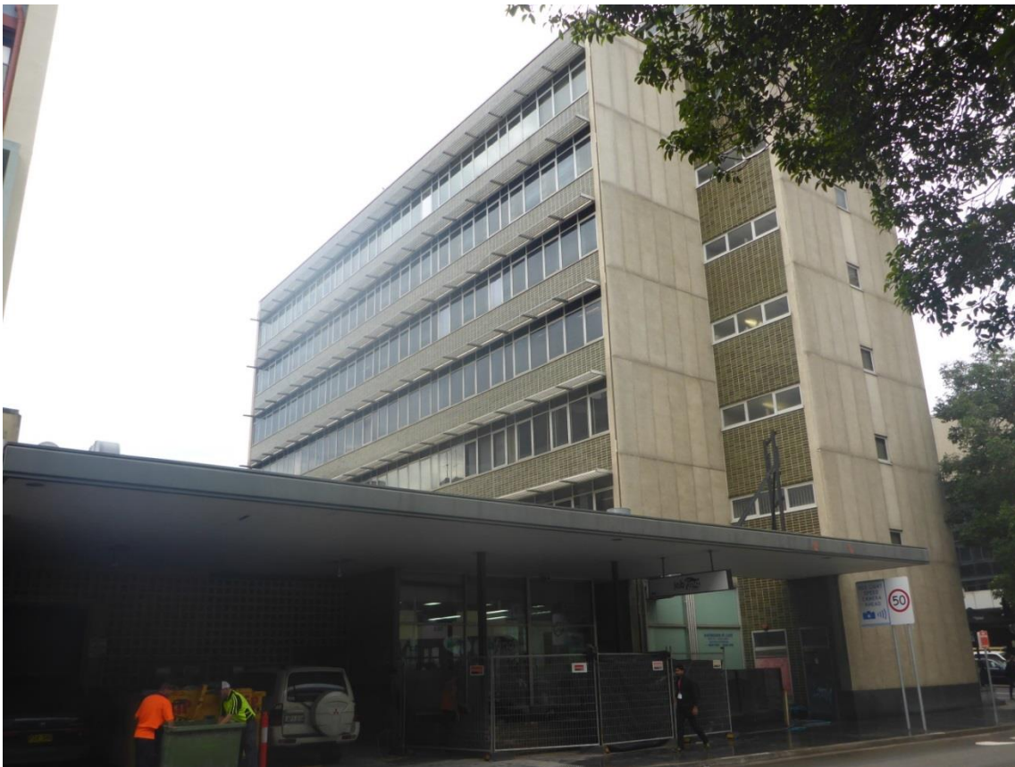
PICTURE 2 – THE WESTERN MARSDEN STREET FRONTAGE AND VIEW OF THE NORTHERN CURTAIN WALL FAÇADE
