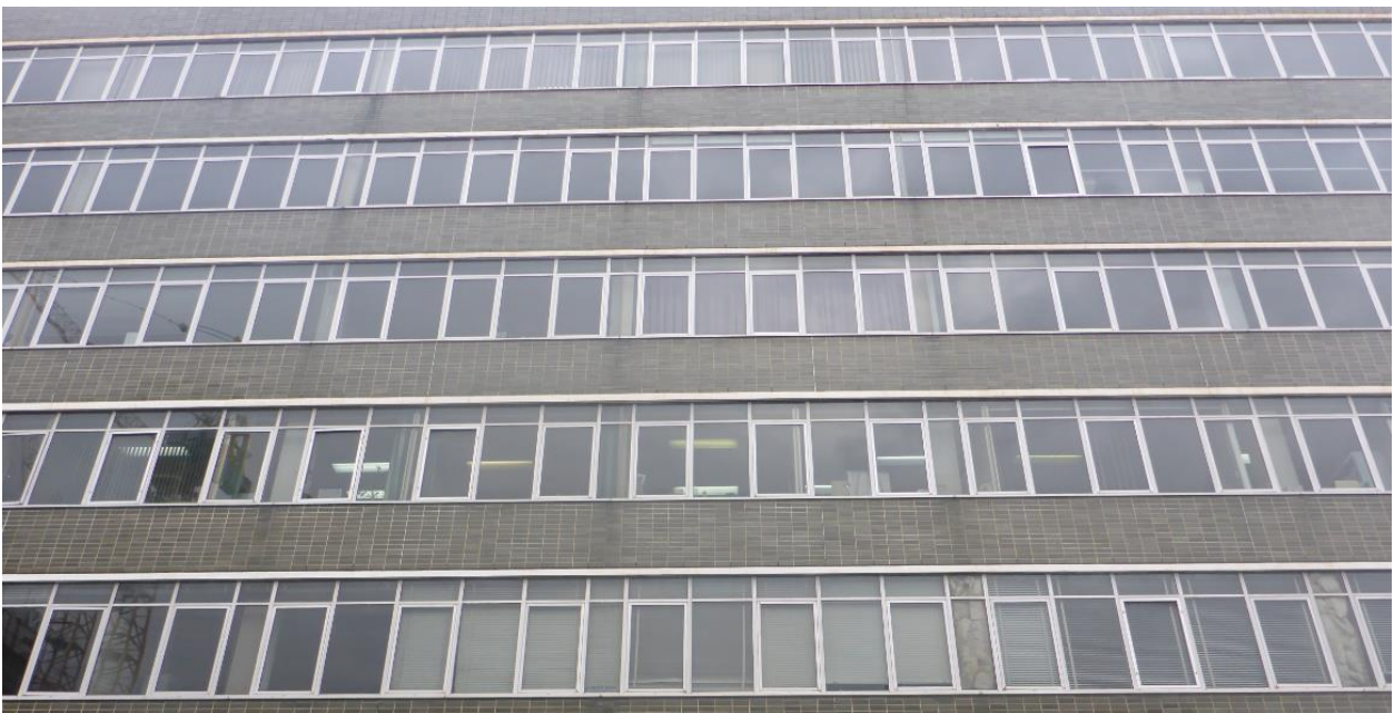
PICTURE 5 – DETAIL OF THE TILED AND GLAZED SPANDRELS TO THE SOUTHERN FAÇADE OF THE BUILDING
