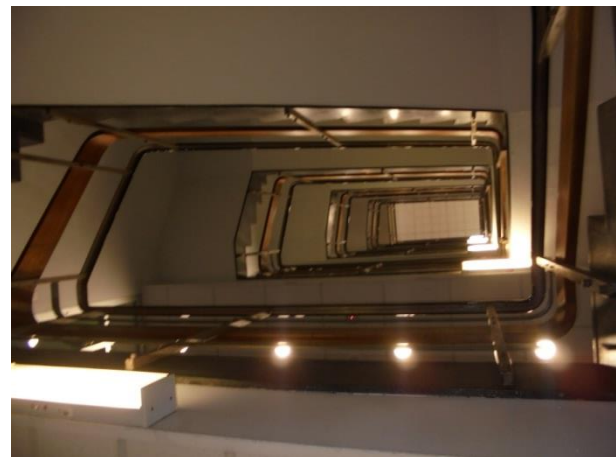
PICTURE 9 – THE ORIGINAL STAIRCASE IS RETAINED
