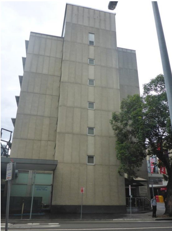
PICTURE 3 – THE WESTERN FAÇADE
