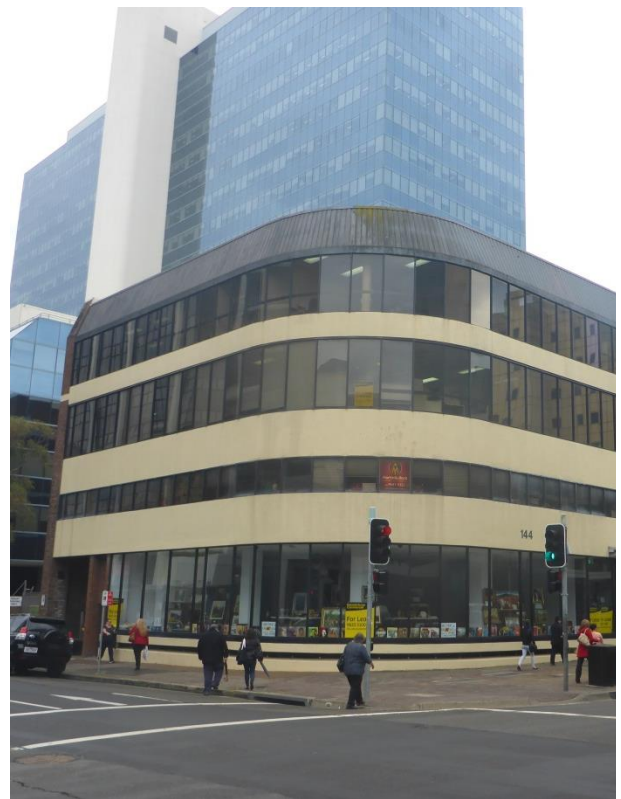
PICTURE 16 – COMMERCIAL DEVELOPMENT OPPOSITE THE SITE ON THE NORTHWEST CORNER OF MACQUARIE AND MARSDEN STREETS
